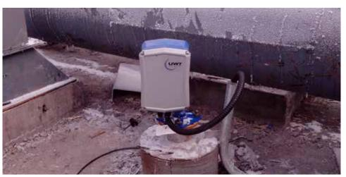
In the preheat decomposition process, the main challenge for any level measurement device are the high temperatures. These are within the section of the grate cooler about up to 600 °C. Whereas the medium temperatures, such as the cement clinker, are about 250 °C to 350 °C. Therefore, the level measurement technology used must be robust and able to meet the high temperature requirements according to the actual working conditions.
